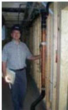
furnace supplies a precise temperature control for excellent energy efficiency. The hot water is supplied by a Rinnai on demand hot water unit and Ken noted that all of the supply pipes are fully insulated, a good idea. Ken noted that drain water
